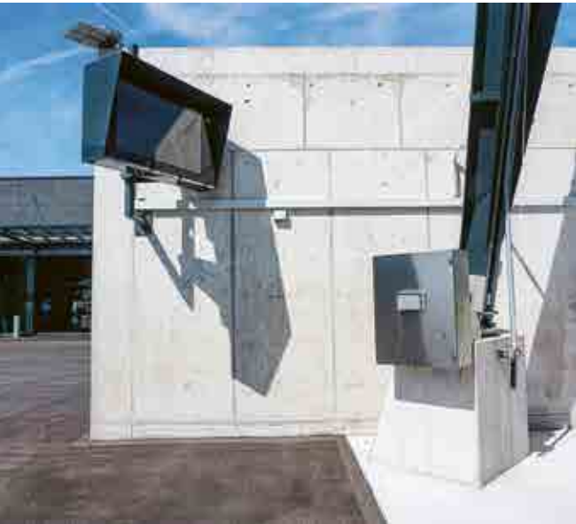
↑ Complete winter services facility with timber silos and brine facility. ↶ The hoppers are controlled automatically via the top-class automatic system. ← The screen helps drivers monitor the filling process.
