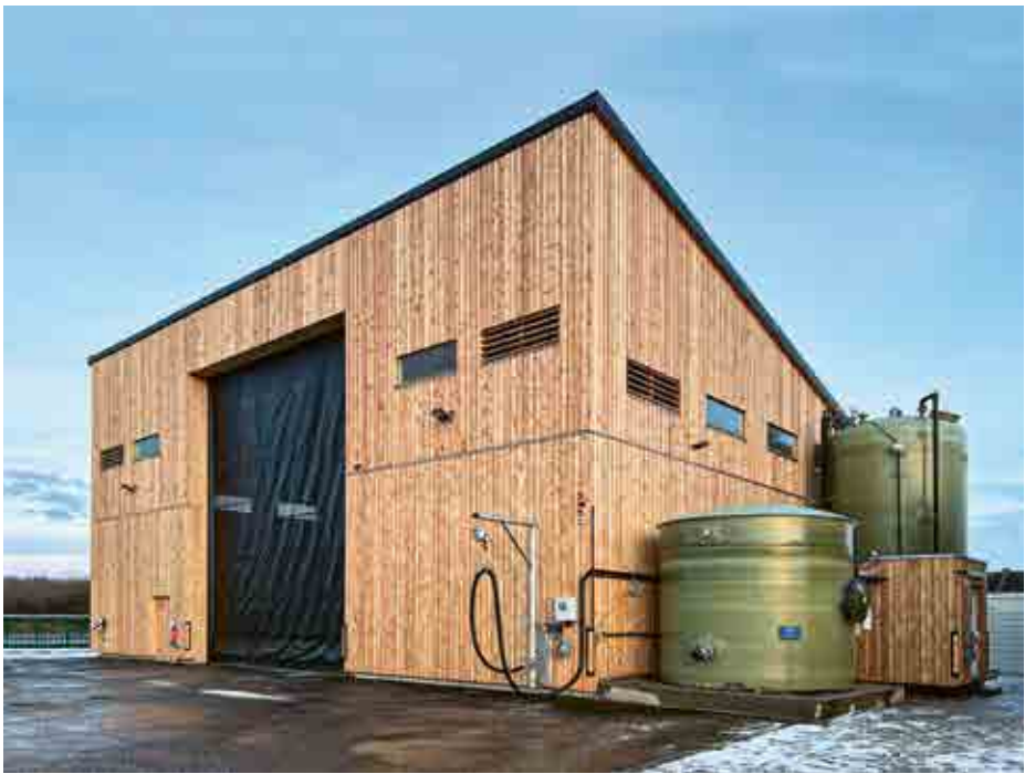
Salt storage depot for 600 m³ of salt with brine facility and technical services room.
