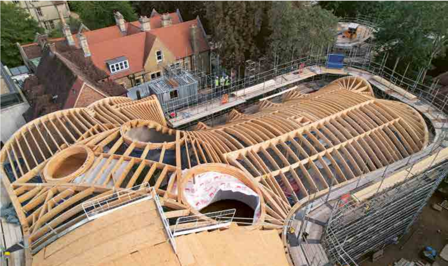
The creative solution for the roof consists of a Free Form with a load-bearing timber structure and conserves embodied energy.
