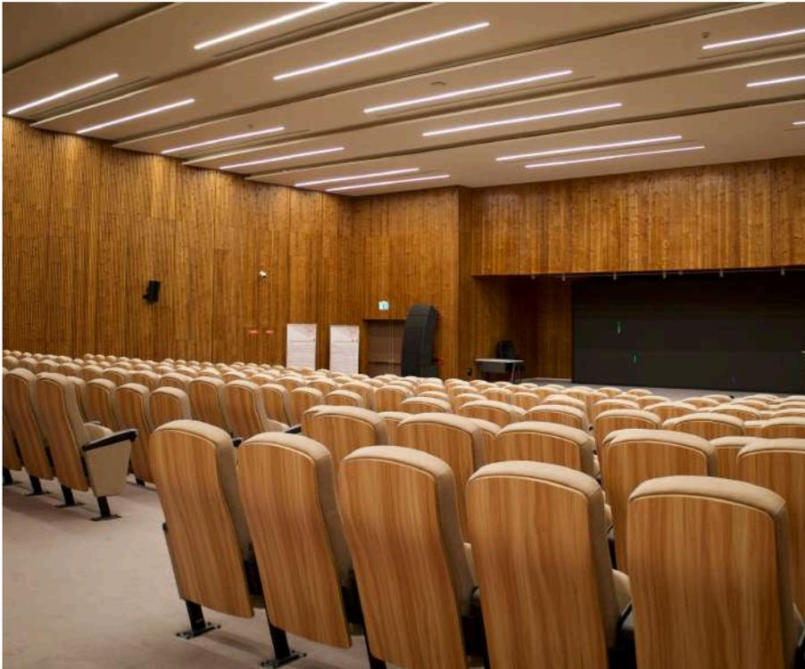
A combination of our paneling profiles: **Triple Shadow 32x140** 3D profile, and **Vivo 19x188**, wide flat profile were used with a supporting acoustical system to clad the auditorium's walls.
