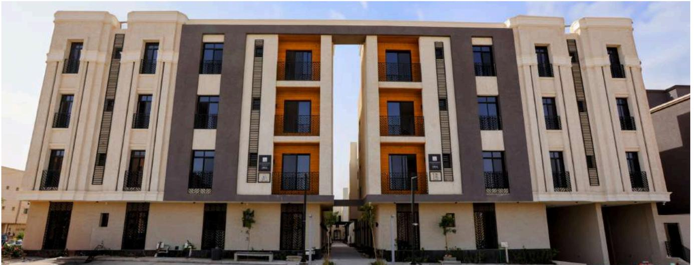
**Luna Vivo 19x188** the wide flat cladding profile, was used for the building's main facade, around the windows. The minimal elegant profile forms a well-defined high-quality wood wall look.
