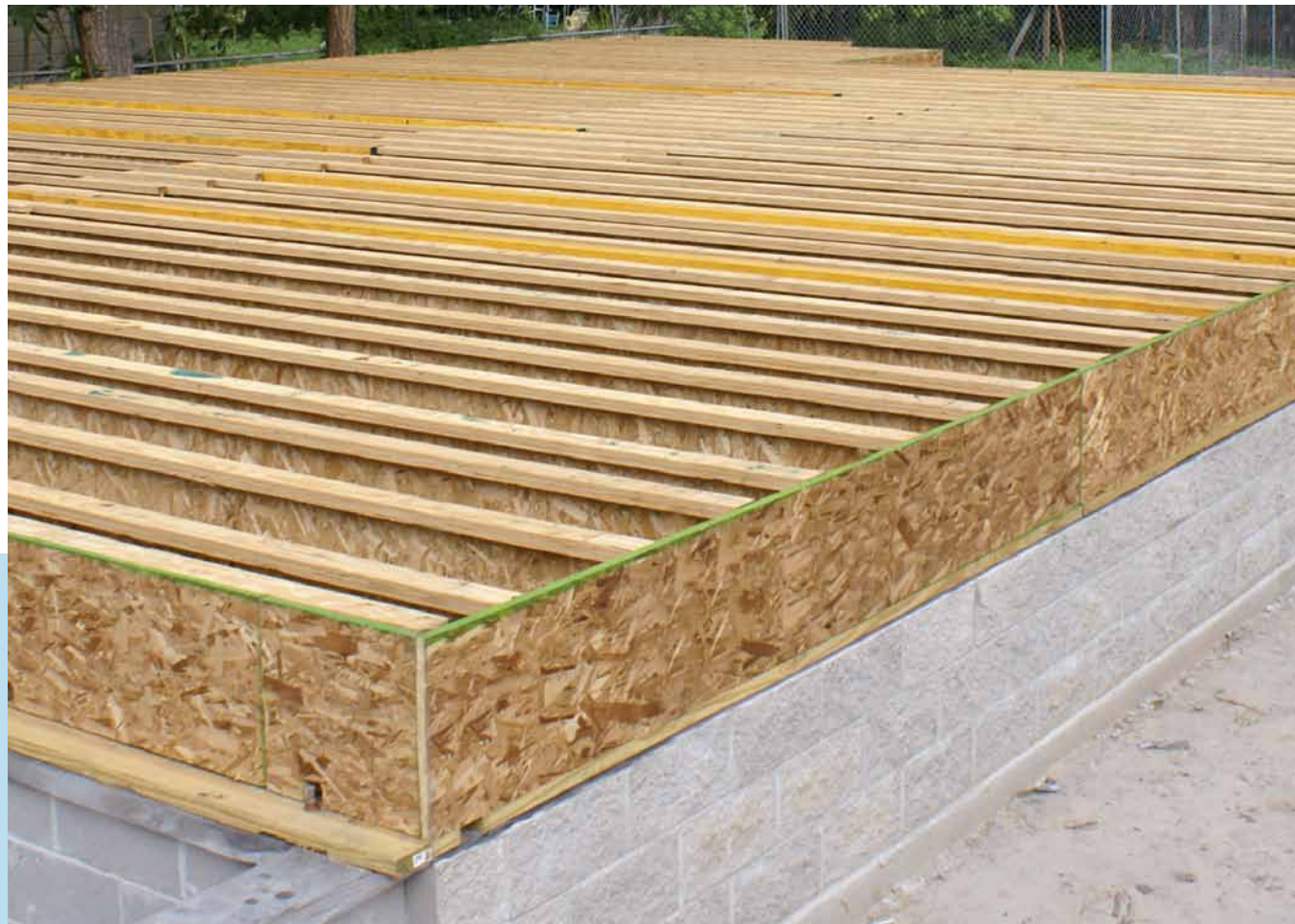
Typical OSB rim board bears fully on the mudsill and is face-nailed into the I-joist flange end and toe-nailed to the sill plate.
