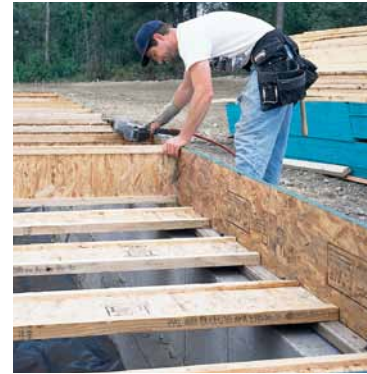
Typical OSB rim board bears fully on the mudsill and is face-nailed into the I-joist flange end and toe-nailed to the sill plate.
