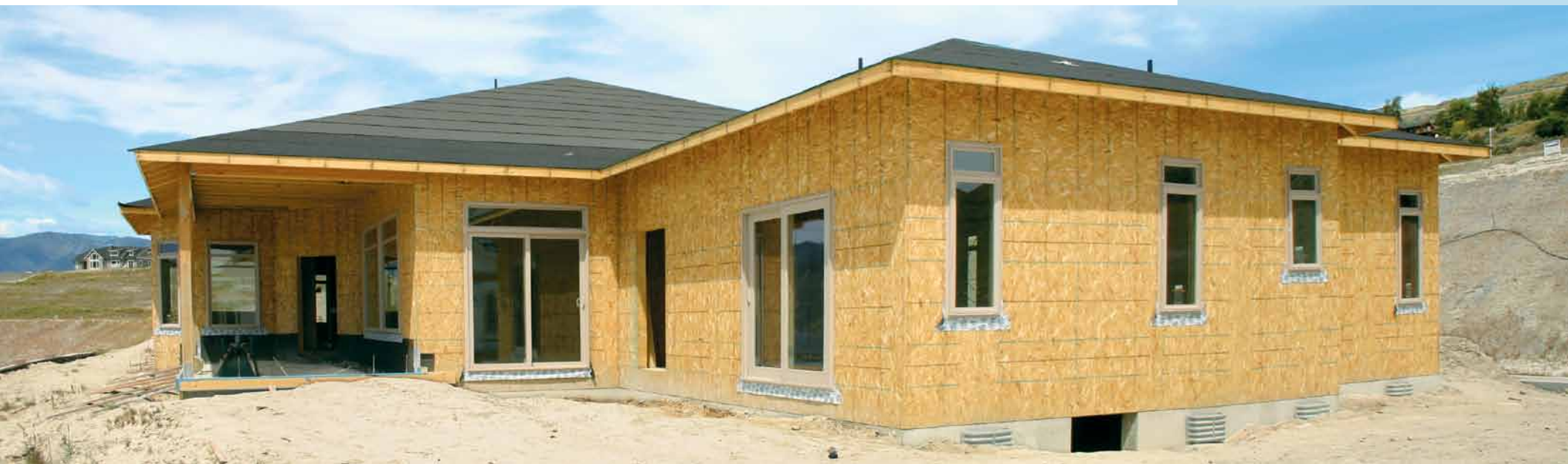
OSB is produced from thin rectangular-shaped wood strands that are formed in a mat.
